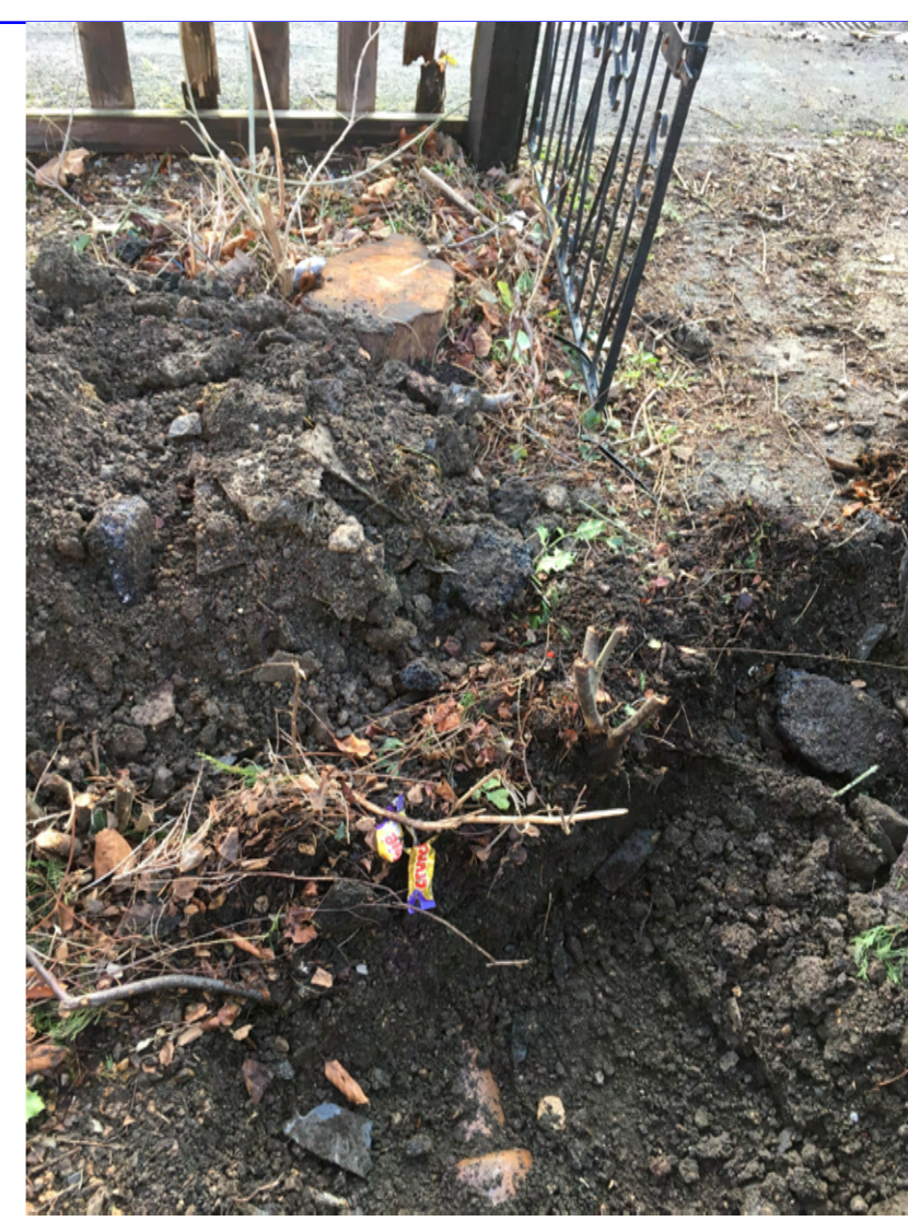
Existing Surface Water Connection
